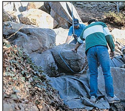
Installing the PondGard Liner
