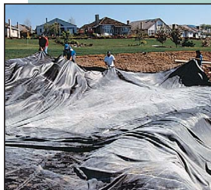
Liner Size Speeds Installation
