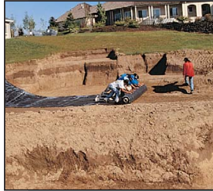
Installing the PondGard Liner
