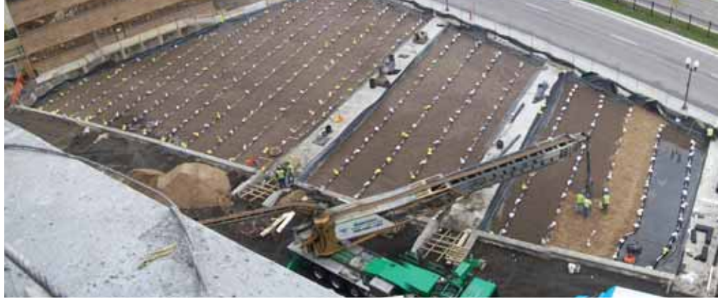
| Aerial view of the stormwater system installation
