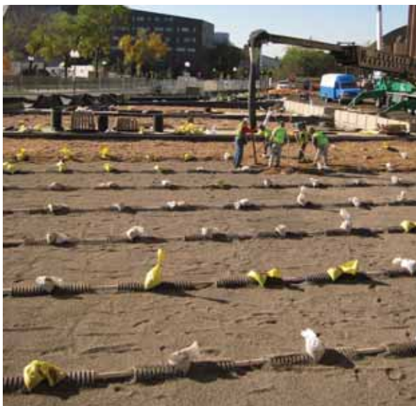
Clean aggregate backfill is applied.
