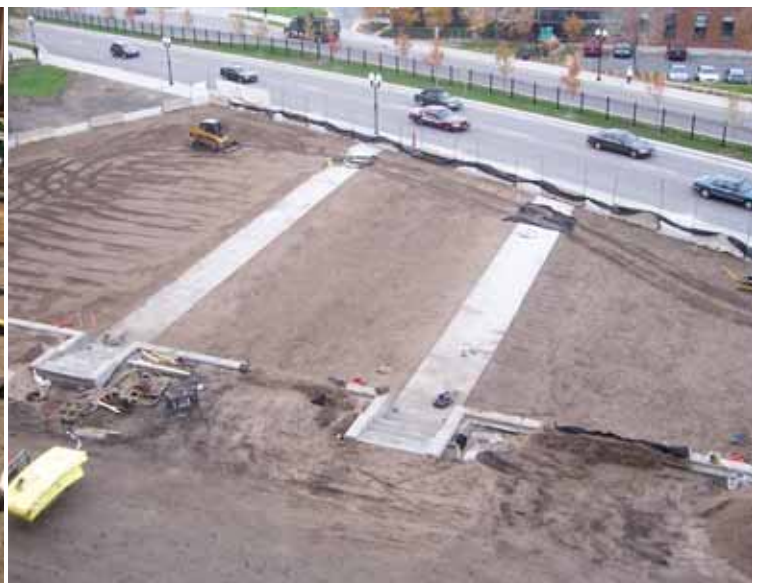
Top grading is completed and prepared for laying sod.
